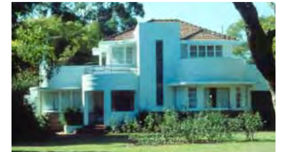
Residence at 32 Genesta Crescent, Dalkeith, O. Chisholm, 1939.
