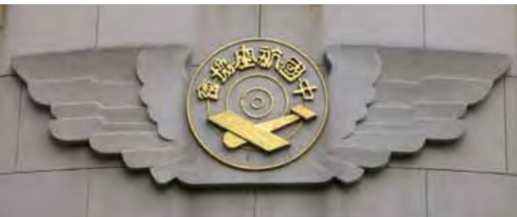
Detail, Civil Aviation Administration Building.
