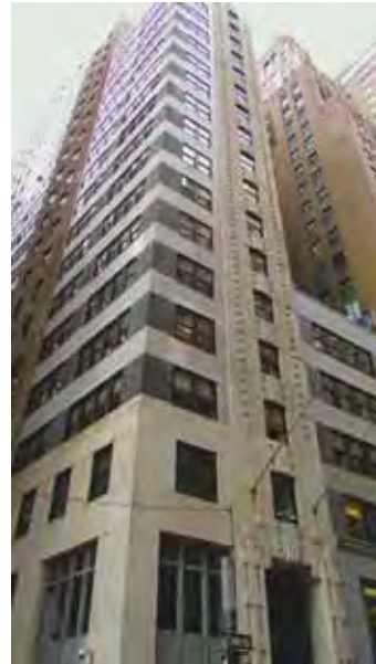
Office tower at 29 Broadway, Manhattan, Sloan & Robertson, 1931.
